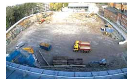
NKS webcams capture the flow of excavation.
