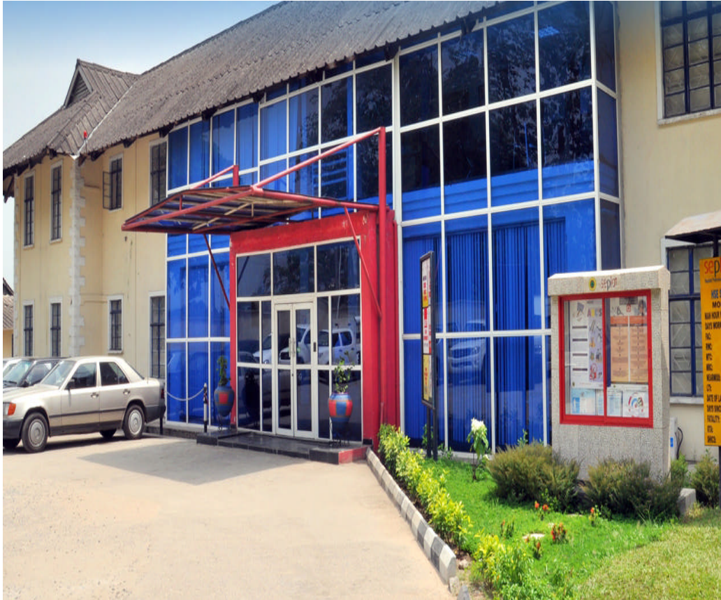
SEPLAT BASE OFFICE, SAPELE
