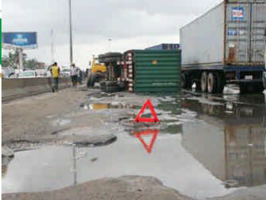
Bad Roads at the main access to Ports
