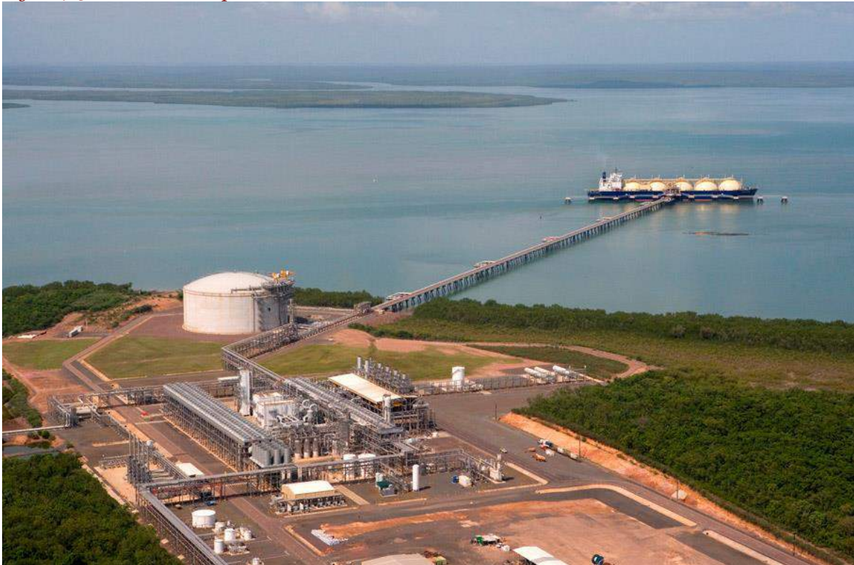
Figure 7.31: Darwin LNG plant in Northern Australia
