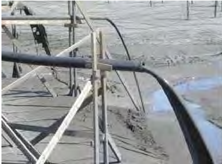
Thickened tailings at Kidd Creek Ontario www.tailings.info/thickened.htm
