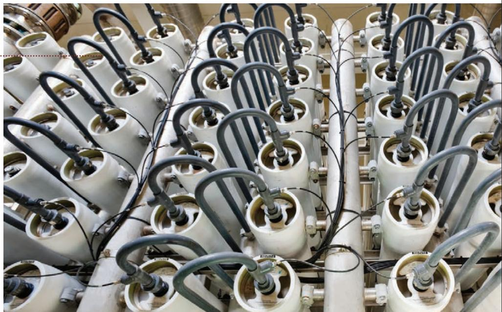
Most desalination plants use reverse osmosis, a process that filters sea or brackish water through a membrane.
