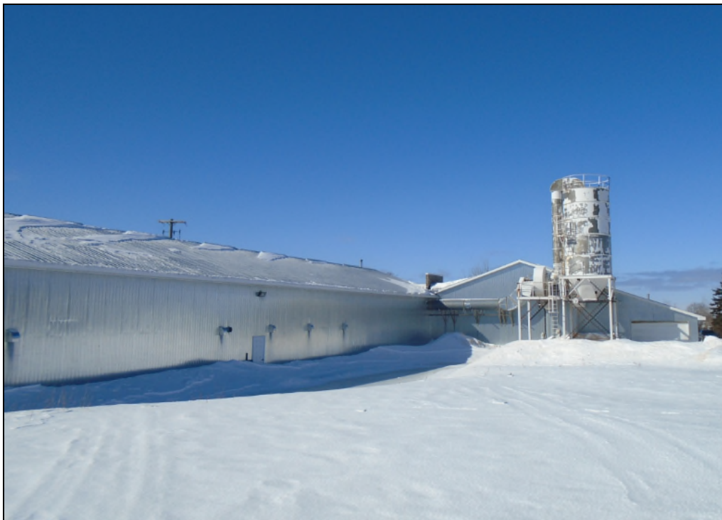
Rear Exterior of the Facility.
