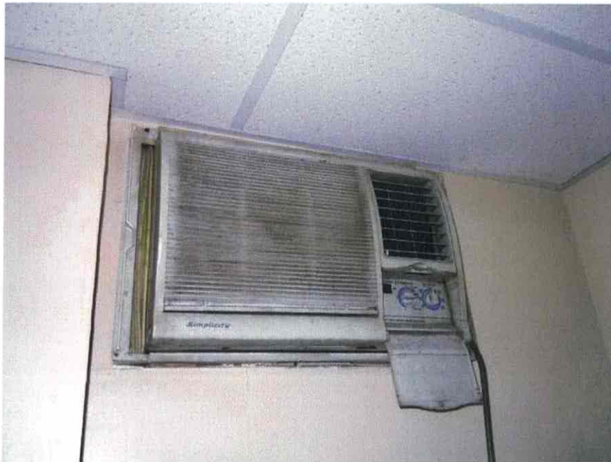
Maintenance Garage / Warehouse – Typical Trough Wall A/C
