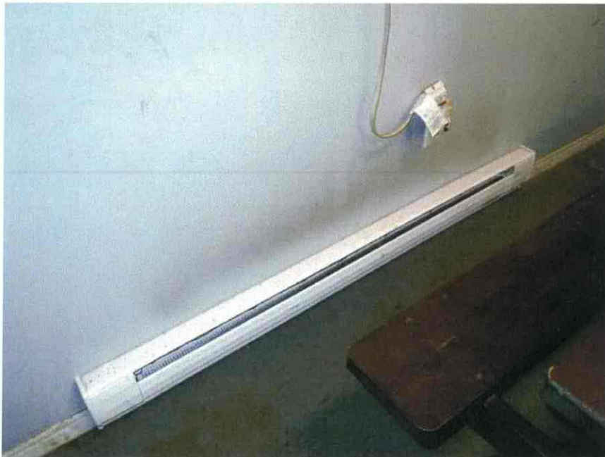
Maintenance Garage / Warehouse – Typical Office & Lunch Room Electric BB Heating
