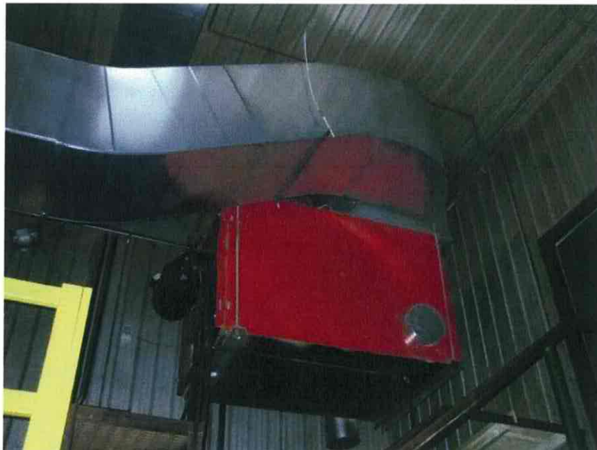
Maintenance Garage / Warehouse – Forced Hot Air Furnace, Waste Oil Burner
