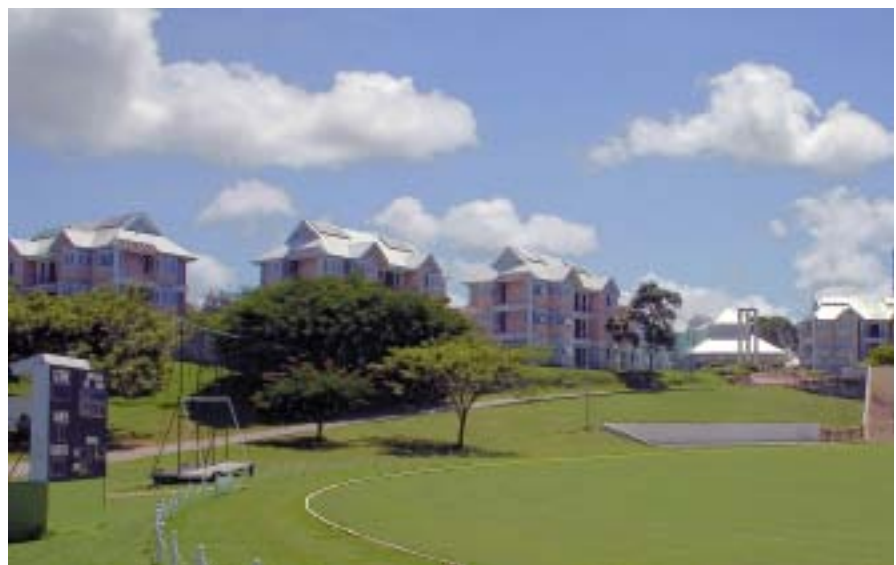
Top: The Sherbourne Conference Centre – one of the most modern facilities of its kind in the Eastern Caribbean.
